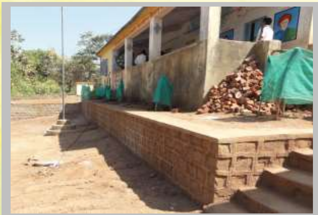
Retaining wall at Bahirampada
